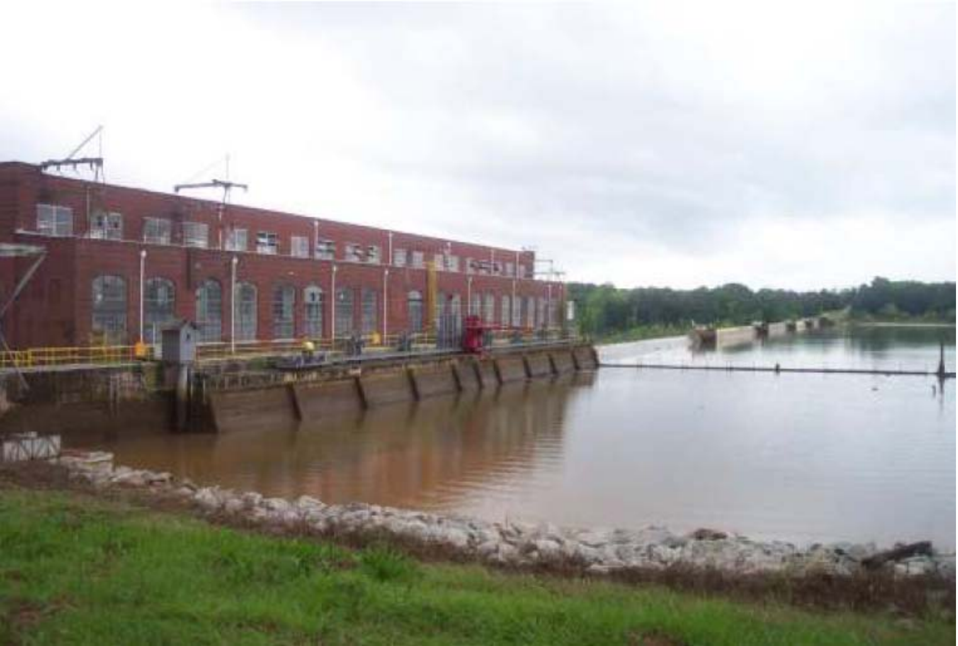
Trash Handling Crane (prior to Drag Rake Installation)
