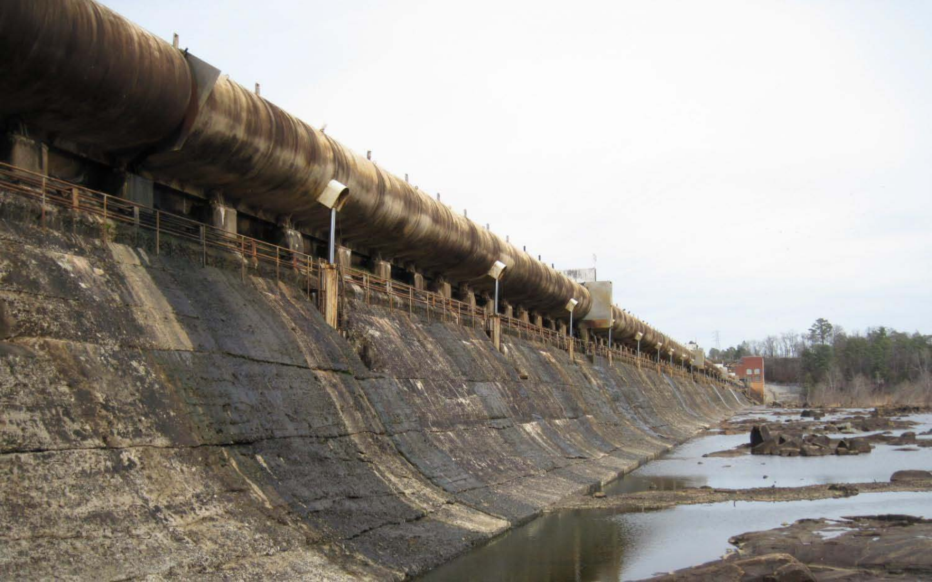
Parr Dam and Crest Gates
